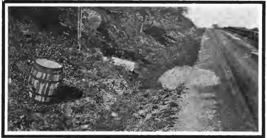
Material for resurfacing and barrels of oil are distributed along patrolled highways in New York
